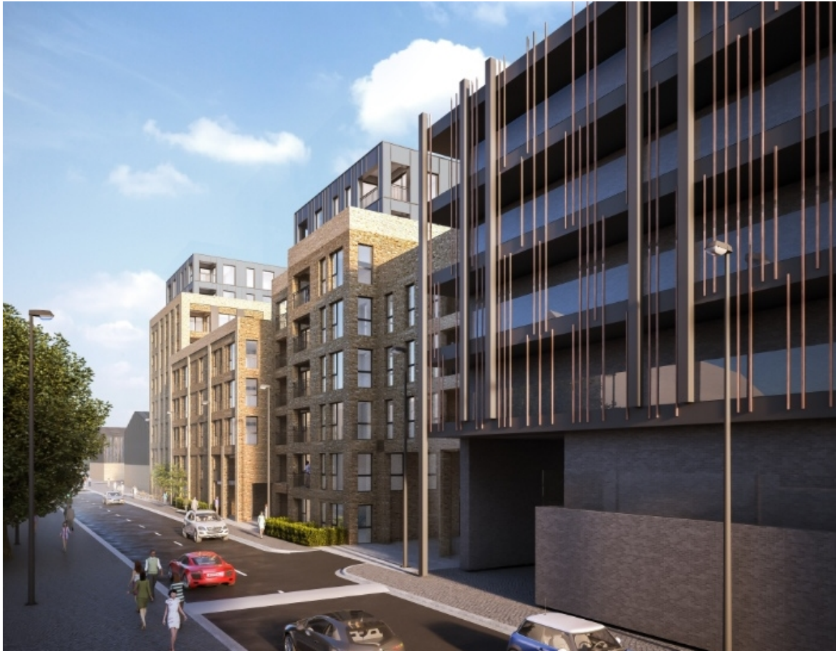
Figure 10 – CGI view of the Thomas Road elevation (Burdett Wharf to the right)
